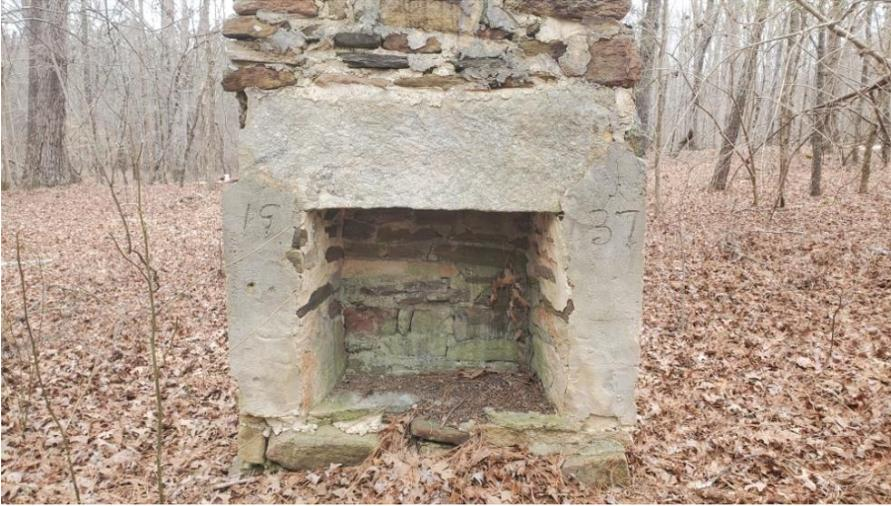
Chimney inscription into concrete, “1937”. Interior includes field stones mortared together.
