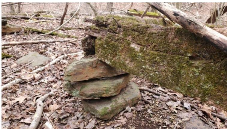
Close up picture of the stone pier foundation and wooden beam.
