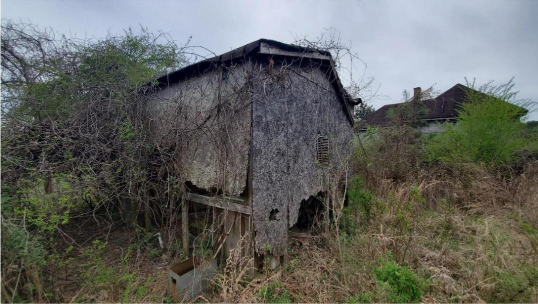
Water and shower shed in front of house. Plywood walls. Deteriorating condition.
